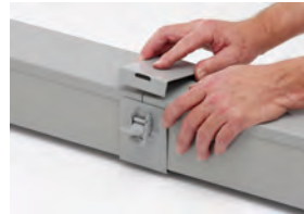
Install outside connector around wireway splice location
