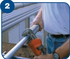
2 With a wrench, tighten the gland nut to compress the Teflon® packing, creating a raintight seal around the conduit.
