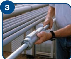
3 Thread the next length of conduit into the other end of the fitting and tighten. You're done!
