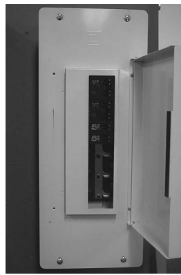
Step #3 Install New HFLCI
