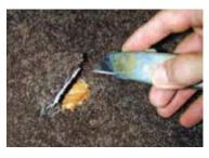
1. Cut a 2-3/8 in. hole through carpeting before using hole saw.
